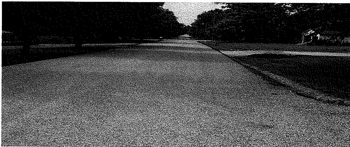
City of Melvern, Kansas - Street condition after improvements
